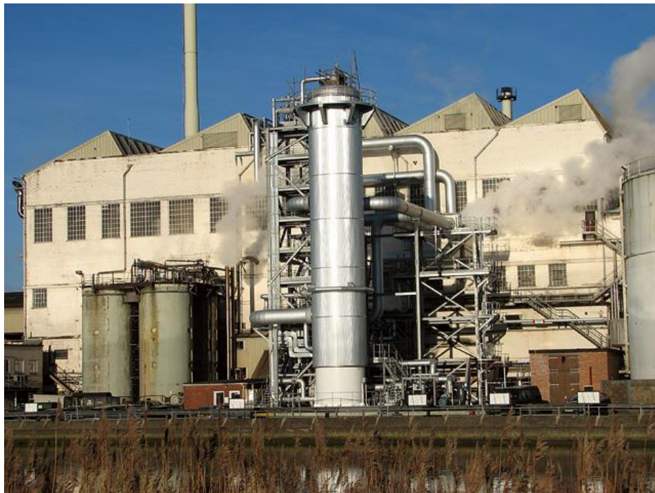
Industrial Evaporator - Photo © Evelyn Simak (cc-by-sa/2.0)
