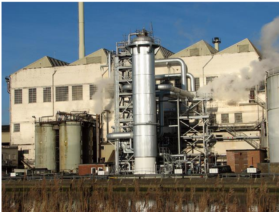
Multiple Effect Evaporator - Photo © Evelyn Simak (cc-by-sa/2.0)
