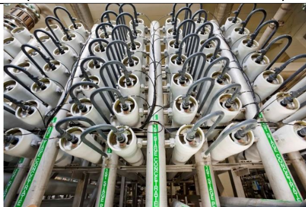
Figure 2: Spiral wound membranes (lateral flow over membrane sheet)
